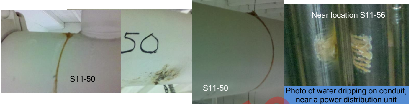
Photos of seepage points discovered
